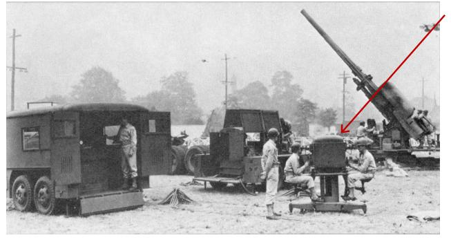
M9 Gun Director - D. Parkinson, Bell Labs, 1943. A revolutionary instrument ! M9's radar tracked incoming enemy aircraft, determined their speed, altitude and direction and then relayed the information to an analog computer that calculated the anti-aircraft gun's trajectory and fuse setting. During one week in August 1944, M9s destroyed 89 of 91 V1 !
